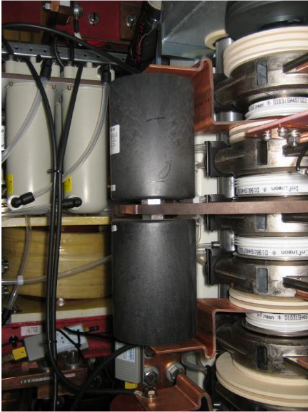
Figure 10–35 Clamp capacitors
