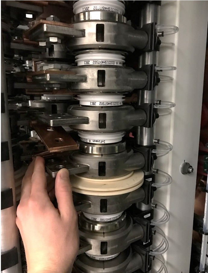
Figure 10–29 Heat sink moved back into position.
