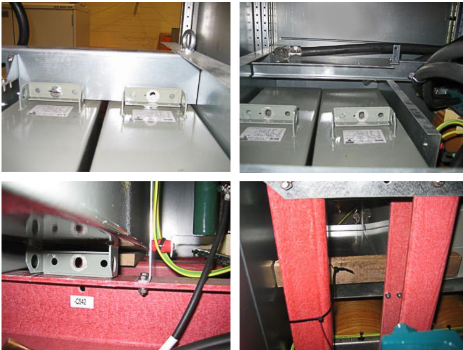
Figure 10–96 Top and bottom views of capacitor
