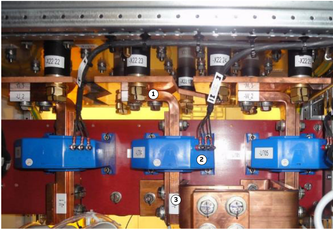
Figure 10–39 LEM current transducers
