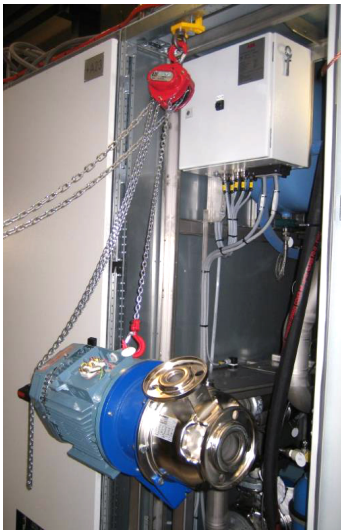
Figure 10–80 Use of chain-block to lift out pump
