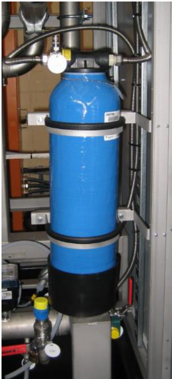
Figure 10–72 Ion exchange vessel (right side: old version)
