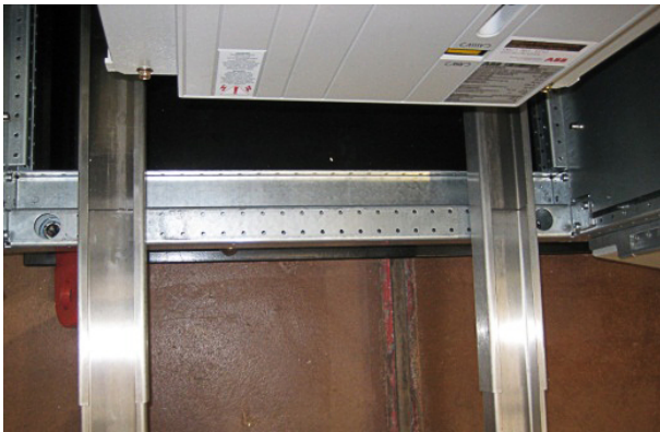
Figure 10–120 Trolley track beams (top view)
