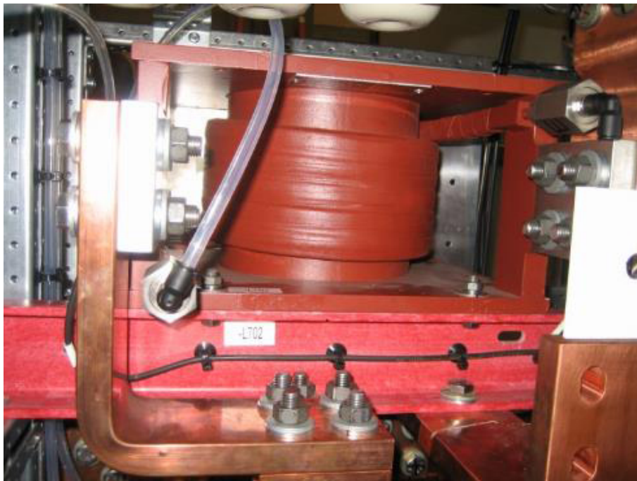
Figure 10–38 Clamp reactor
