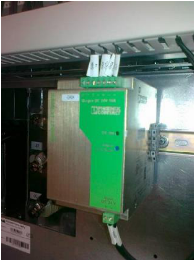
Figure 8–18 DC/DC converter Quint-PS-24DC/24DC/10
