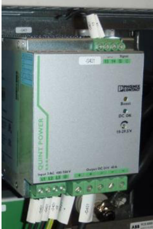
Figure 8-16 AC/DC converter Quint-PS/3AC/24DC/40
