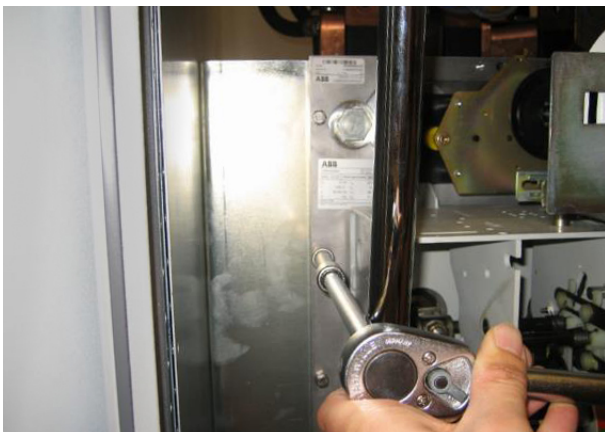
Figure 10-124 Unbolting the GEB
