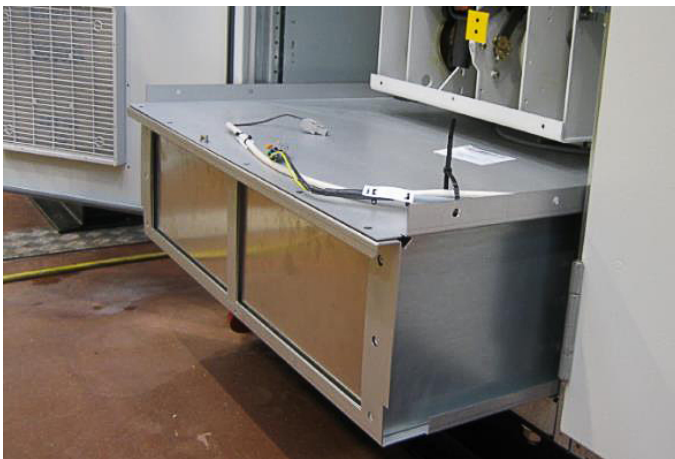
Figure 10–111 Fan drawer below the GEB
