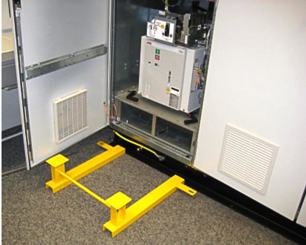
Figure 10–119 Support by reactor replacement kit
