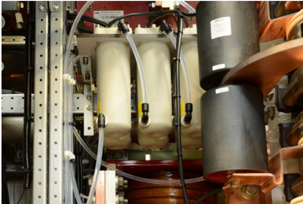
Figure 10–37 Clamp resistor
